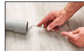
Feed End of Tape Into Conduit
