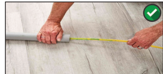
To protect from insulation damage, Always pull the wire from conduit at 180° angle.
